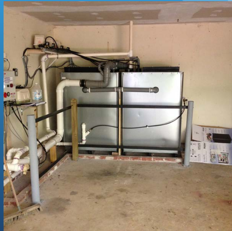
MBR with nutrient removal and advanced disinfection
